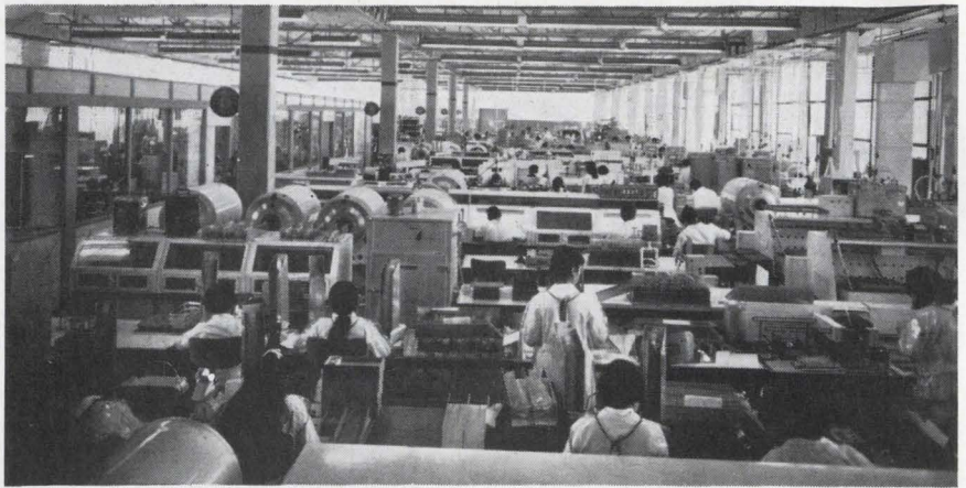
Assembly. Electronics S.A., a Mexican affiliate of M.V. Philips, turns out semiconductor devices at this modern plant in Toluca.
