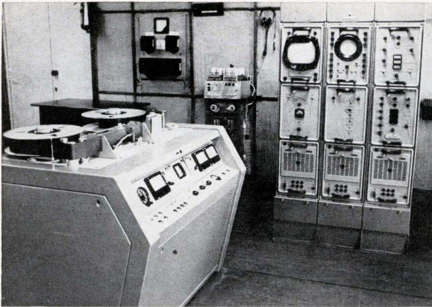
New Soviet video tape recorder in Leningrad studios is similar to Ampex VR-1000.
