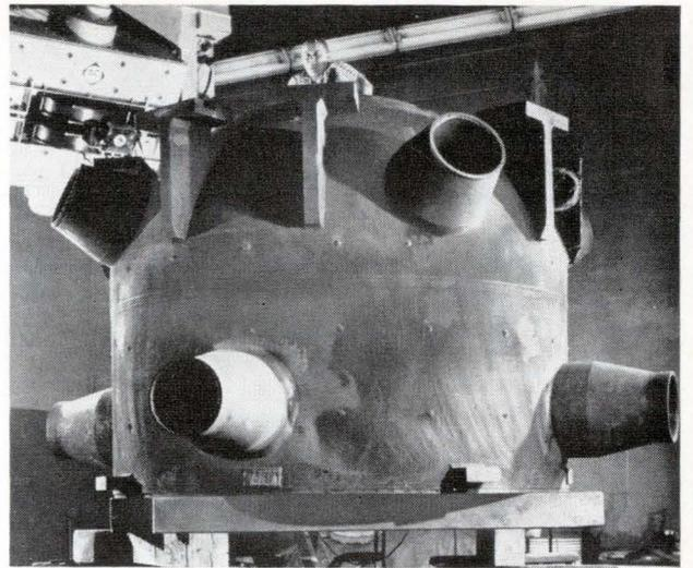
A flaw in a weld of the bottom portion of this atomic reactor can not be allowed.
