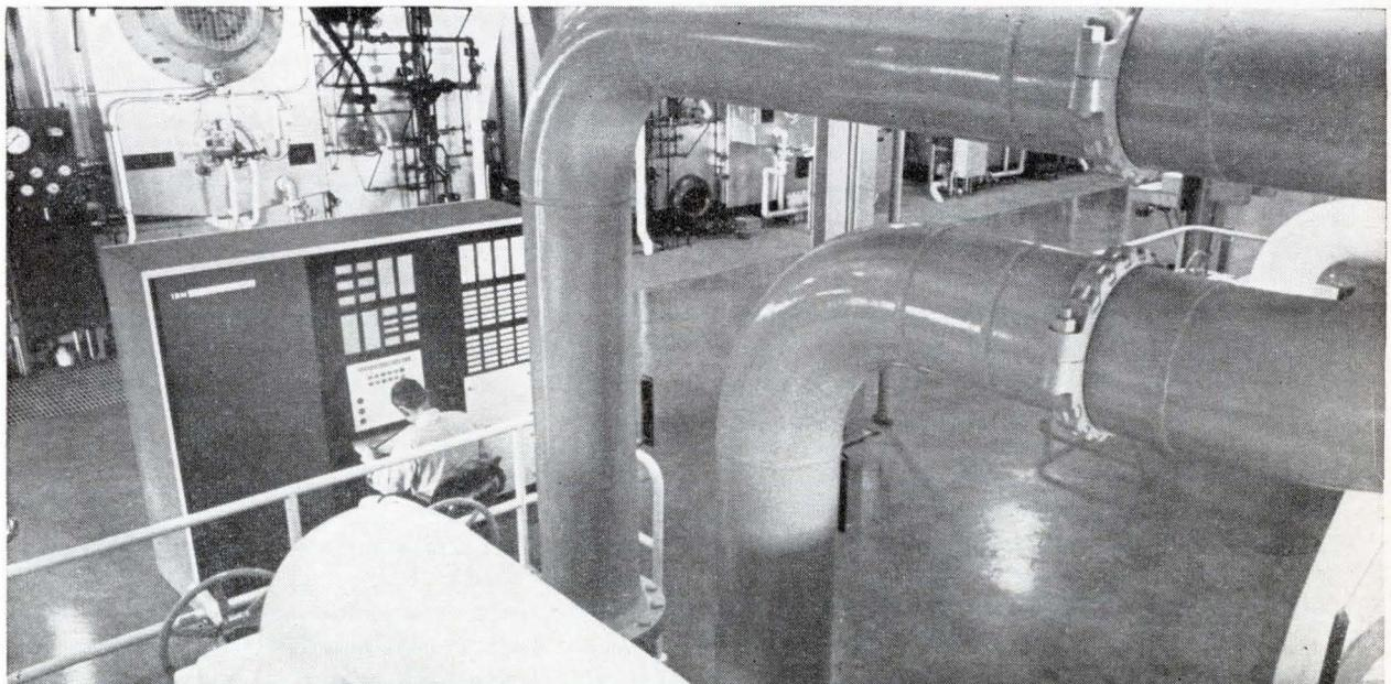
**Model 1800 computer**, made by International Business Machines Corp., is designed specifically for direct digital control of industrial processes such as electric utilities' steam generating plants.
