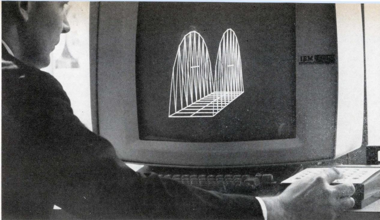
**Three-dimensional image of a bridge**—generated by a mathematical model stored in an IBM System 360 computer—can be examined and manipulated by instructions to the computer. Using the keyboard at right, the operator can display the bridge from different angles and can make the image—or parts of it—larger or smaller.
