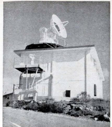
FSP-16 radar, built by RCA, starts tracking missiles at 2,000 feet.
