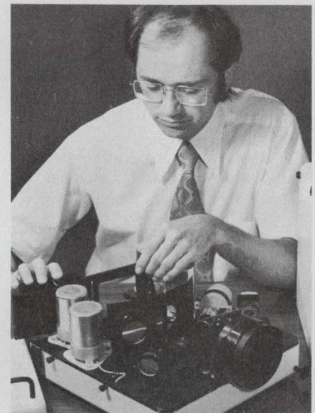
Hand-held holography is possible with this lightweight holographic camera, developed by Dr. Donald H. Close at Hughes Research Laboratories.
