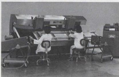
**Computer automated production system** — wire routing, component placement and wire wrapping.
