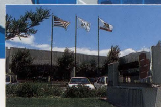
Samsung's U.S. Headquarters in San Jose includes Engineering, Marketing, Sales and Administration and also boasts state-of-the-art R&D and Class I manufacturing wafer fabrication.
