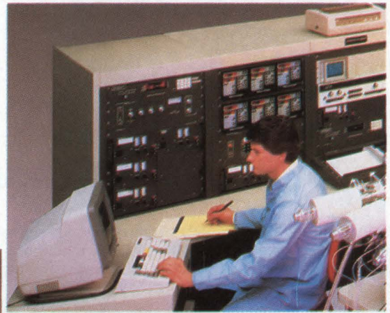
CONSOLE AREA MOUNTS THE KEPCO POWER MANAGERS
