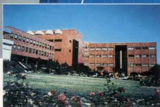
Samsung's sophisticated manufacturing facility at Bucheon employs internally-developed Advanced CMOS and Bipolar processes.
