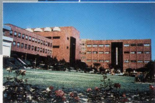
Samsung's sophisticated manufacturing facility at Bucheon employs internally-developed Advanced CMOS and Bipolar processes.
