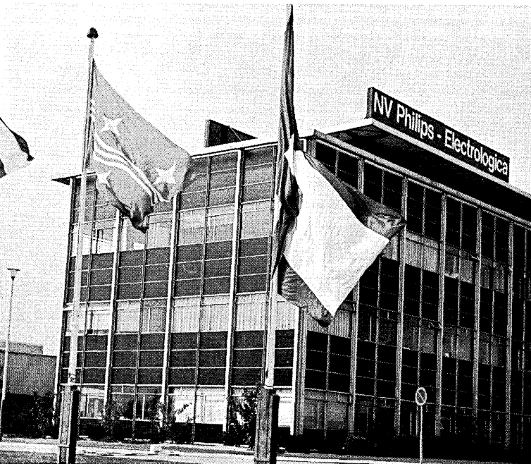
A corner of the Apeldoorn (Netherlands) complex of buildings where 12,000 Philips employees turn out the P1000 series of computers. This multinational giant has additional major manufacturing centers in Germany, France, Belgium, and Sweden.
