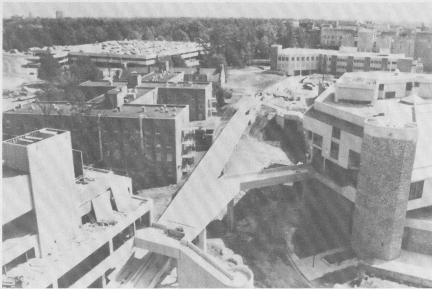
Figure 5: When Duke University Hospital expanded, older facilities were connected with new ones by means of an AGT.
