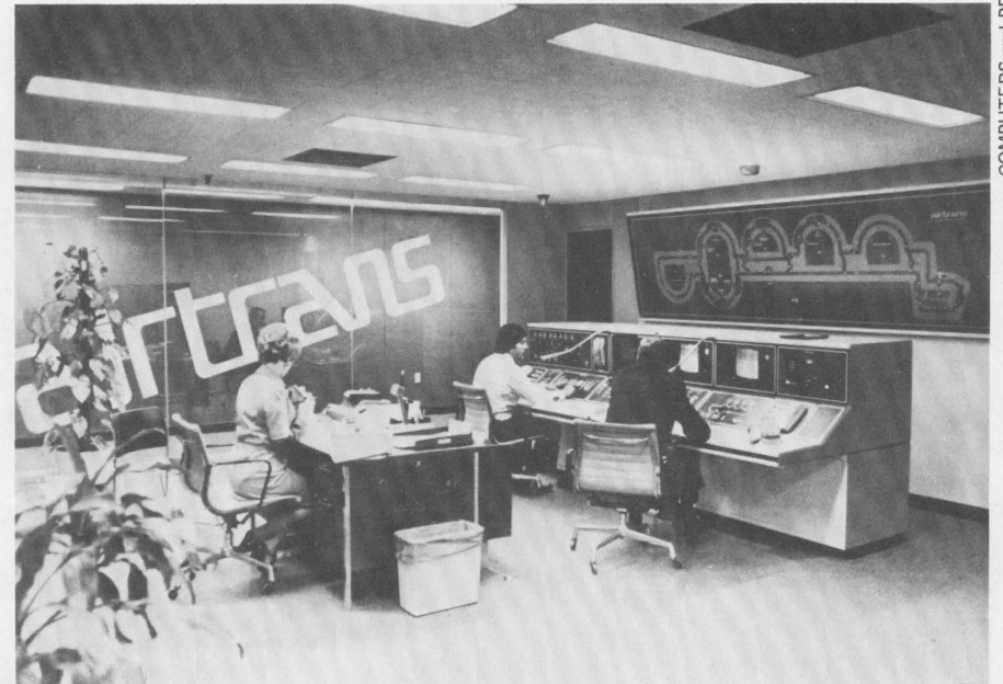
Figure 4: This control center at Dallas-Ft. Worth airport keeps track of 53 stations and 67 vehicles.
