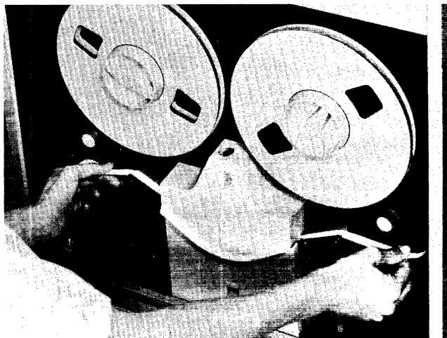
Figure 2-7. Tape Alignment
