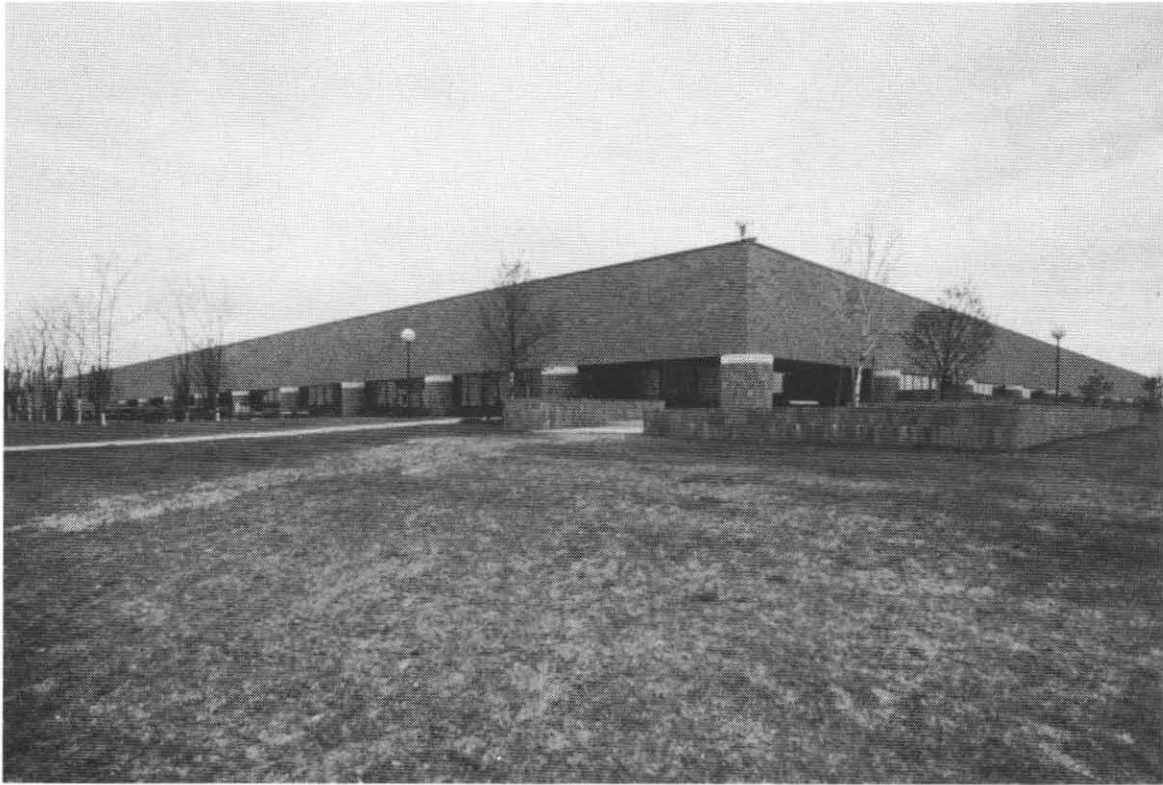
DIGITAL Facility, Hudson, Massachusetts
